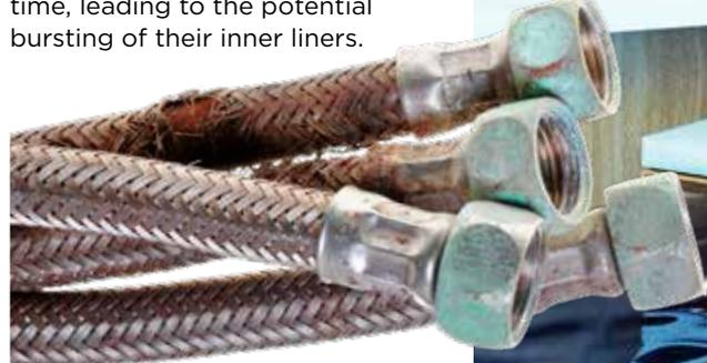
Current flexi water hoses have a short shelf life and unless you have installed the latest Abey 'Polyamide' Hi Class Easy Hooker, you could get into deep water. Abey Hi Class Easy Hookers offer the highest class of rust protection and a massive 15 Year Abey Rust Resistance Warranty.
